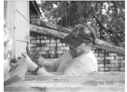
Paul attaching the wall of the new shed.
