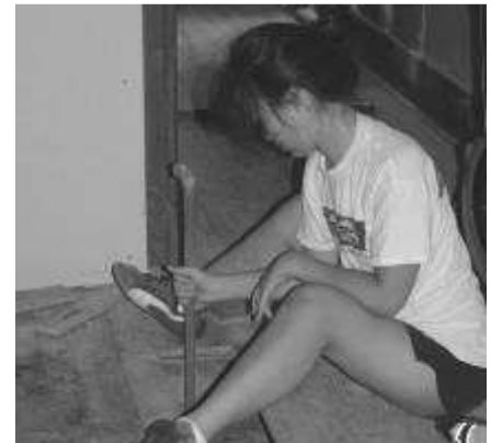
Jennifer prying nails from the old floor.
