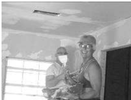
Bill and Gayle working on house number one.
