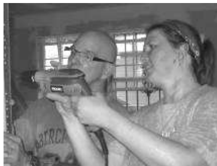
Jenny and Bill installing corner bead at house number one.
